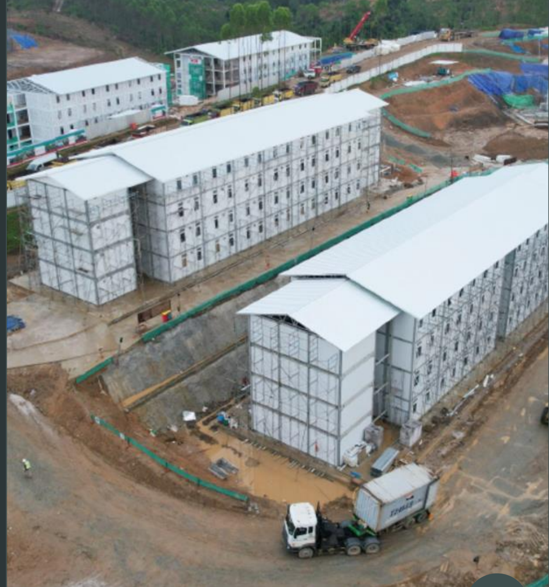
Housing compounds for construction workers
