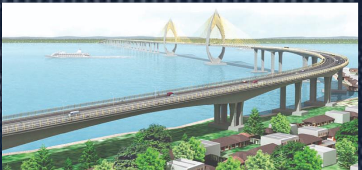
Toll Bridge – Balikpapan Bay Offered for Investment
