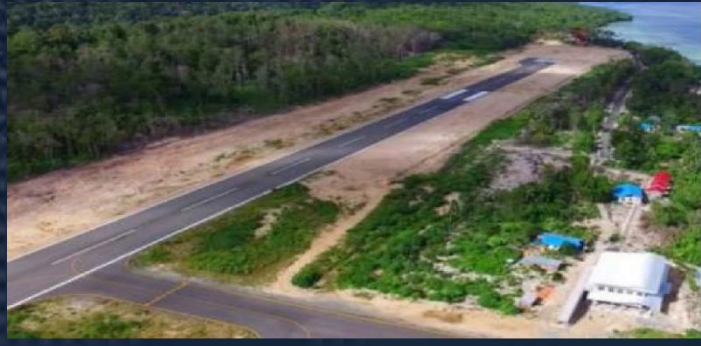
Maratua Island Domestic Airport Operational
